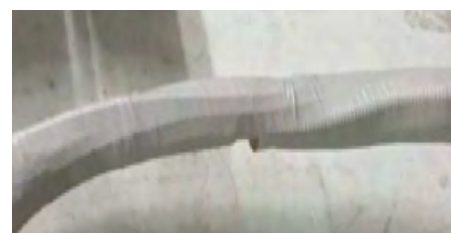
Figure 7.8B - Final Insulated Piping Bundle with Drain Hose Orientation
