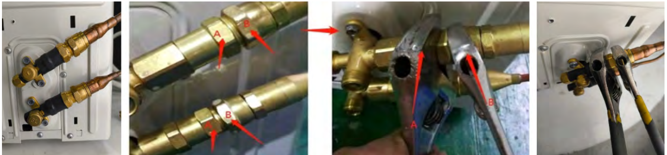
Figure 8.4D - Two-Wrench Tightening (Remarks A & B)
